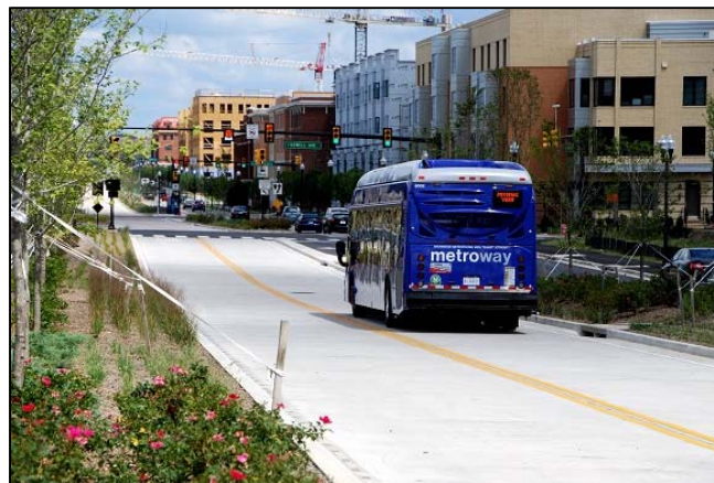
Busway in Virginia. Photo: Alexandria, VA Transportation & Environmental Services
